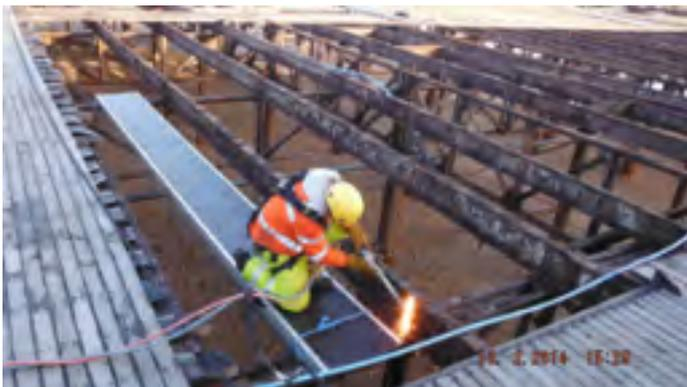
*Above: Works underway in 2014. Slicing through deck beams. Image © Ramboll*
