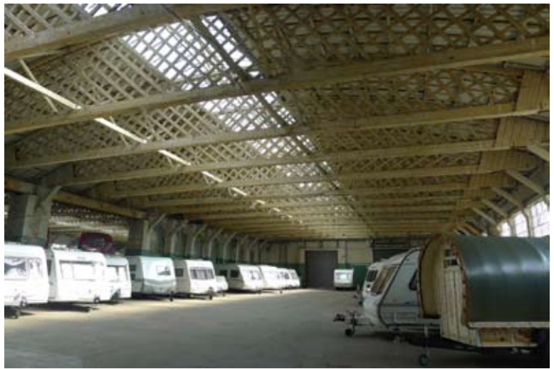
Fig 4. The interior of the central General Service Shed (© English Heritage, photograph: Clare Howard)
