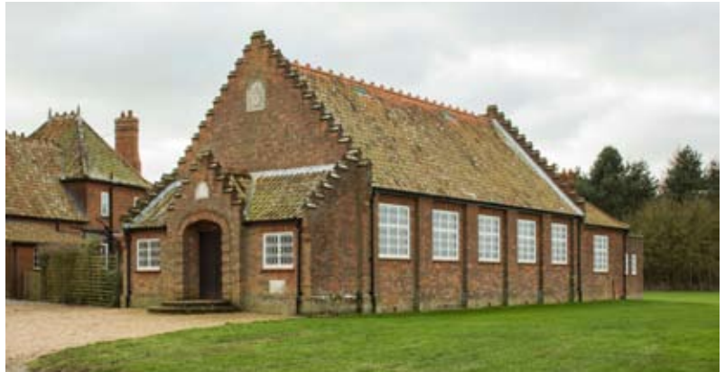
Fig 3. The Memorial Hall of 1929 at Salle (Norfolk), recently listed at Grade II. Designed by the Norwich architect Edward Boardman, its crow-stepped gables echo those of the school alongside, built half a century earlier. Historic England
