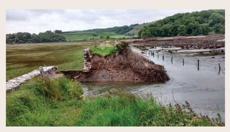
Photograph showing the breach in the bank and where the phases of construction can be seen. Credit: Judith Doyle
