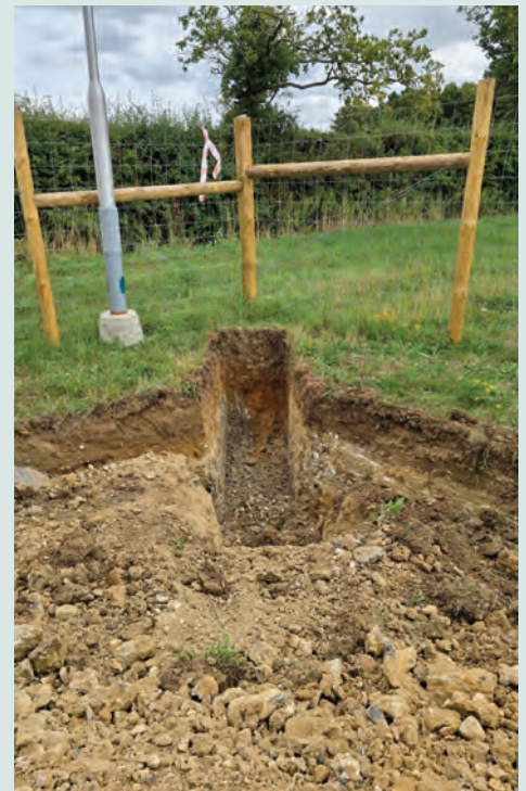
Perimeter fence and CCTV cable trench. Credit: Pre-Construct Archaeology
