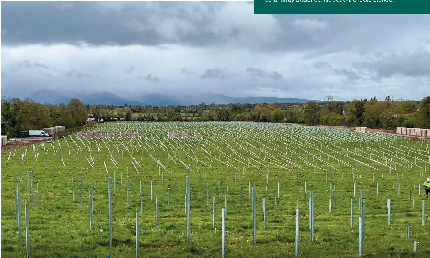
Solar array under construction. Credit: Statkraft
