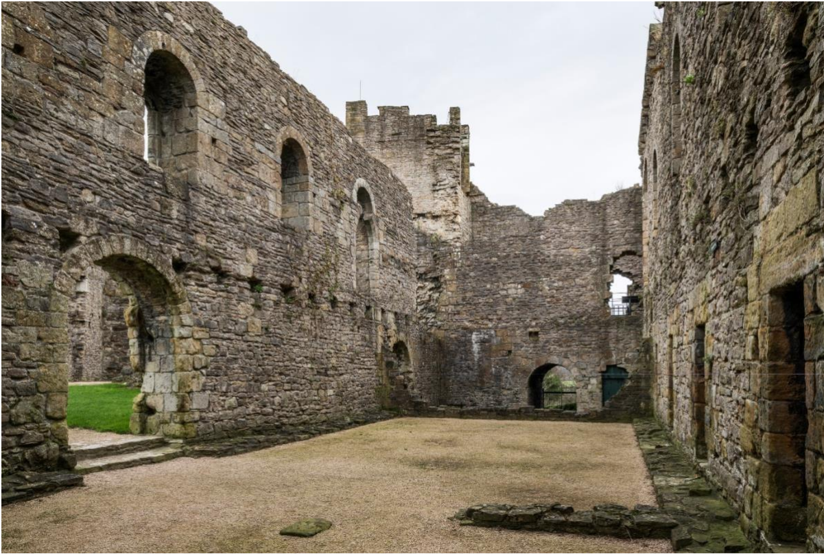
Figure 2. Scolland's Hall, looking east. The put-log holes on the left wall mark the level of the first floor, the photograph being taken in what was, in the late 11 th century, a ground-floor undercroft. © Historic England Archive
