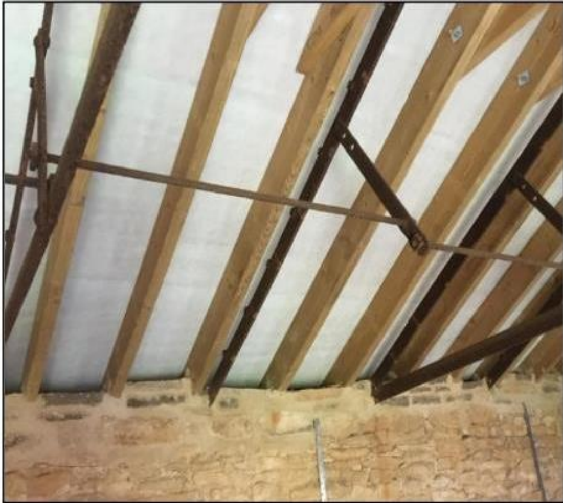
Rafter frame with rafter post attached to adjacent trusses by connecting rods. Building B. Photo D Hill
