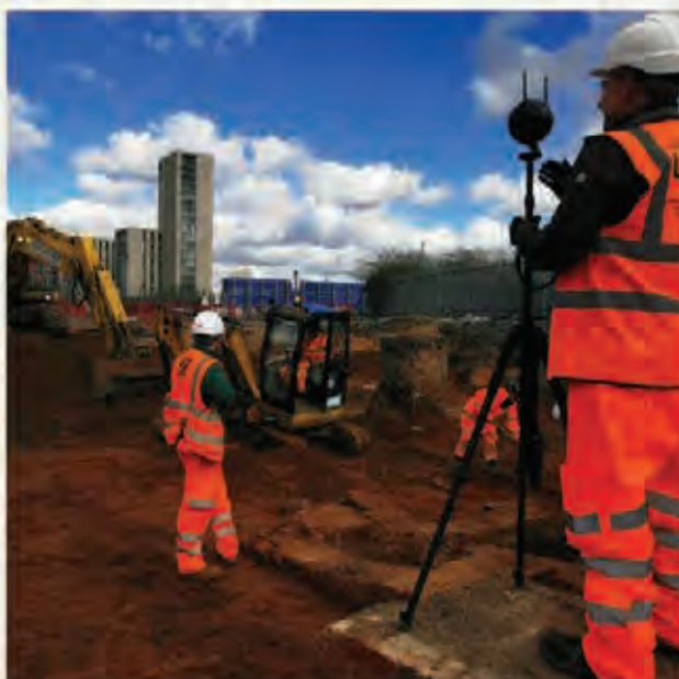
360-degree video camera setup to record excavation. Credit: Visualising Heritage, University of Bradford; © HS2 Ltd
