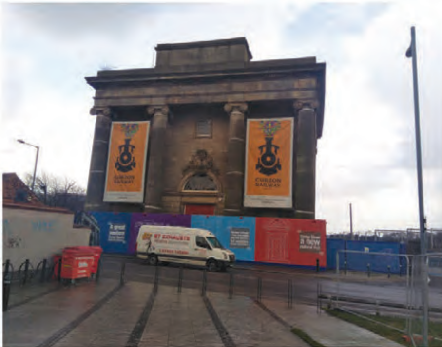
Grade I listed London and Birmingham Railway terminus Principal Building, Old Curzon St. IR38 (monitored for movement and cracking; influencing the design of the new station). Credit: Stonebow Heritage. © HS2 Ltd
