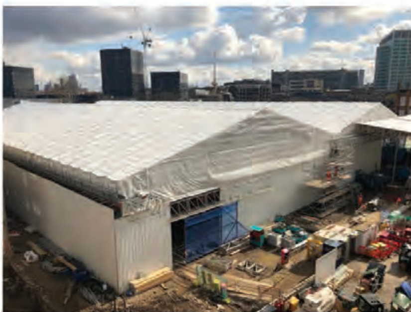
Encapsulation structure over the big dig at St James's Gardens in Euston designed by Costain Skanska JV. Credit: Caroline Raynor, Costain Skanska JV, © HS2 Ltd
