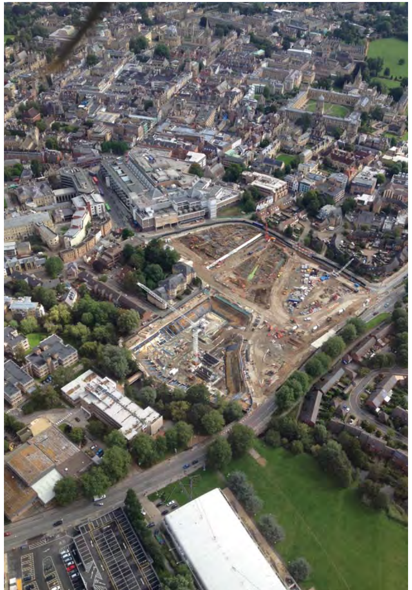
Aerial shot of the site and western part of historic Oxford. Credit: a friendly helicopter pilot
