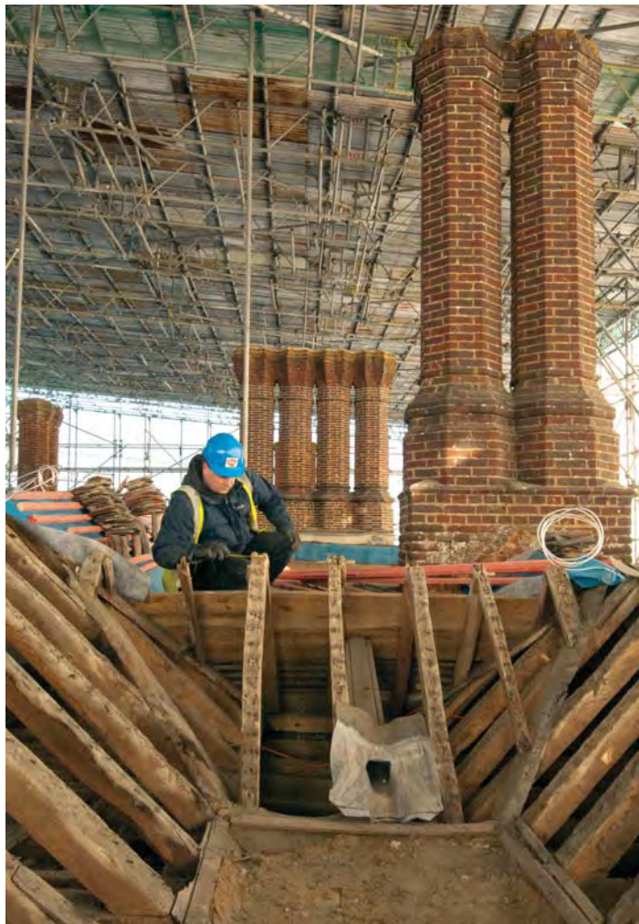
Knole House building recording. Credit: MOLA
