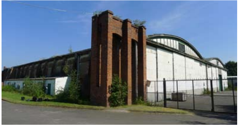
Fig 3. The southernmost General Service shed (© English Heritage, photograph: Clare Howard)
