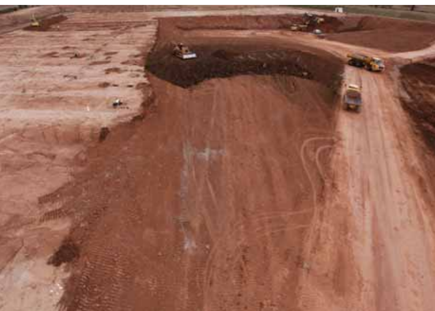
Commercial archaeology has generated much new data about areas of the UK which were little studied 20 years ago. At this quarry archaeological investigation revealed a previously unsuspected Romano-British landscape on the Warwickshire claylands, where little previous work has occurred and which is not particularly susceptible to aerial or geophysical survey. Photograph: AerialCam
