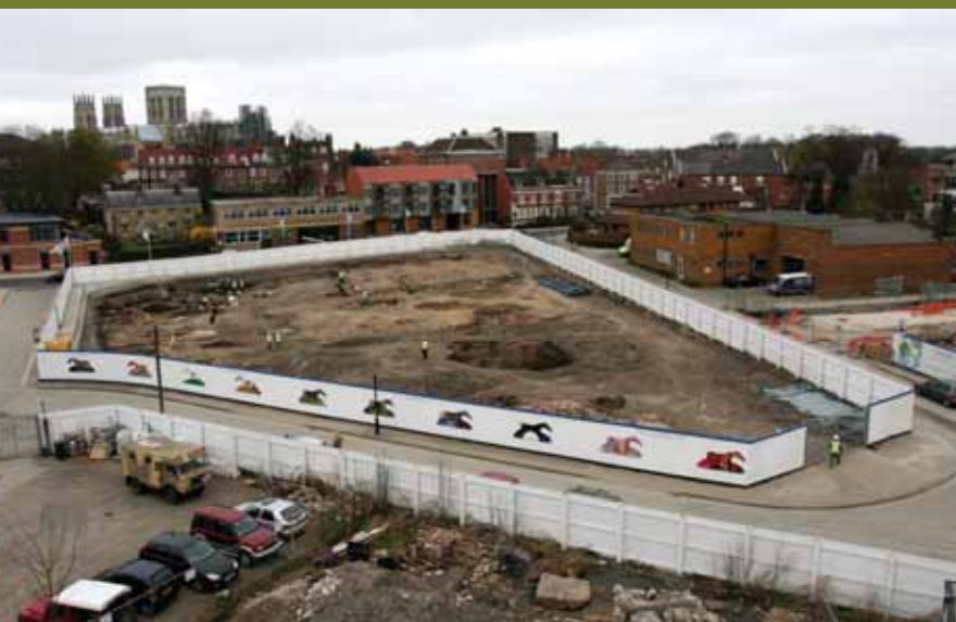
Looking across the main Hungate excavation area in 2009
