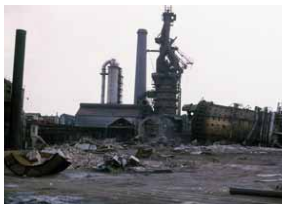
◀ The blast furnaces at Stanton, Derbyshire, being demolished in 1976. © David Crossley
