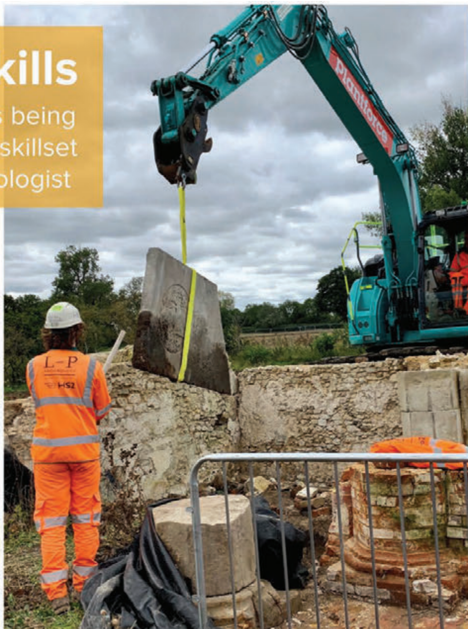
Lifting supervisors to overseeing lifting on site. Credit: L – P Archaeology; © HS2 Ltd
