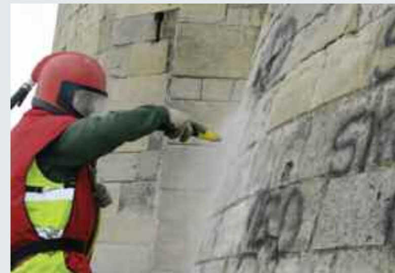
Graffiti removal in York, Clifford's Tower © to Yorkshire post
