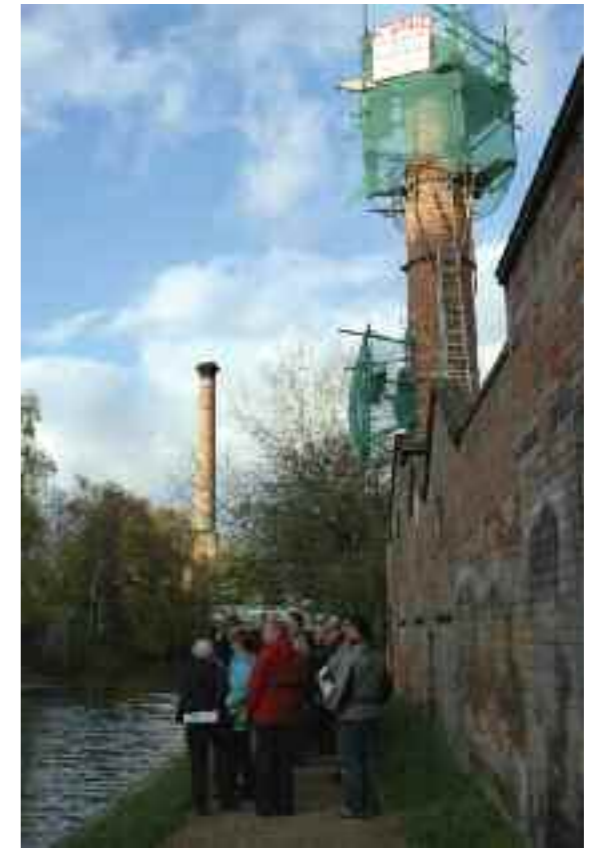
Industrial buildings seminar tour of the textile mills at Long Eaton in the East Midlands
