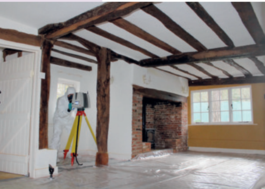
Laser scanning the chemically-damaged 14th-century timber-framed cottage
