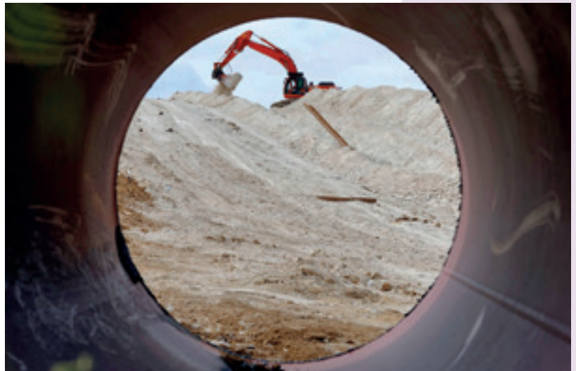
Pipeline project, Kent (Photo: Adam Sandford, Aerial Cam)
