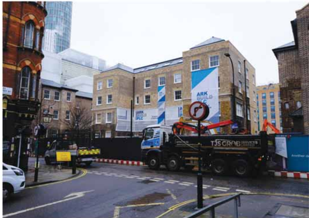
Retained workhouse. Credit: Icenl Projects
